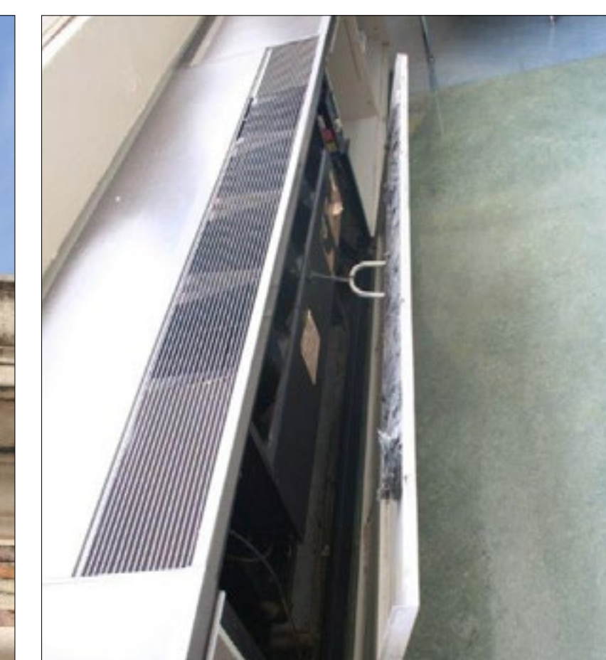
TYPICAL UNIT VENTILATORS
