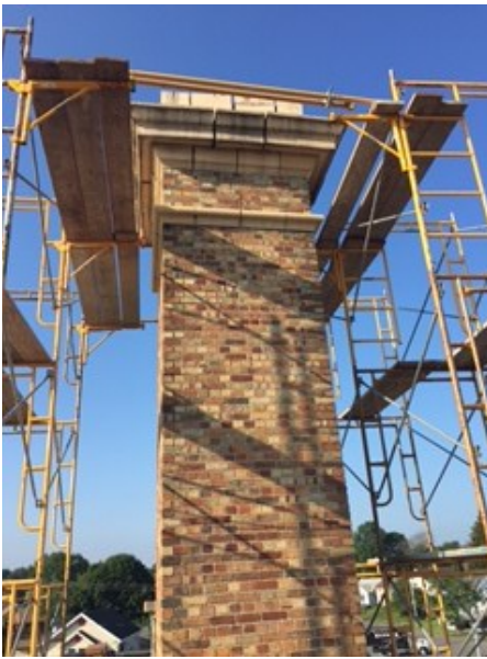
Re-pointing & repair of the stone coping and chimney
