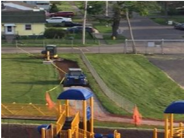
Sidewalk Excavation and Base
