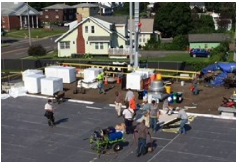
Roofing system & rooftop ventilator replacements over the 1932 and 1965 building wings.
